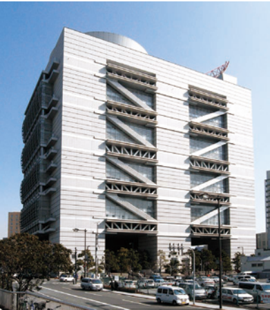
Conference center (application of steel Unbonded Braces)
